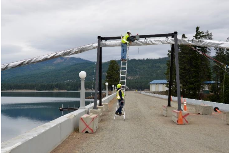
Fig.4. Simple over road tube hanging structure.
