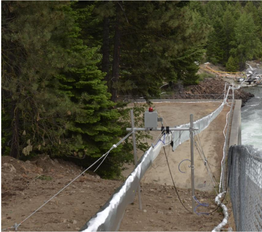
Fig 2. Simple temporary support stand for over land tube section
